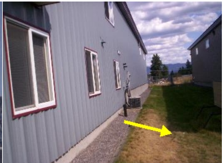
Right side of building - proper perimeter grading
