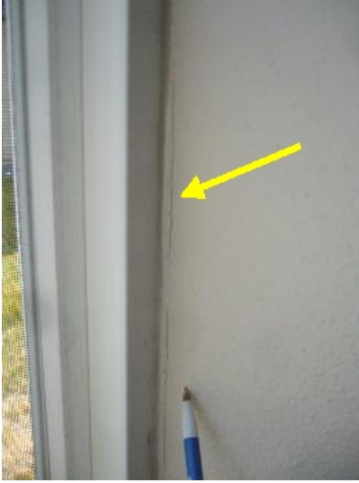
As maintenance caulk around windows as needed
