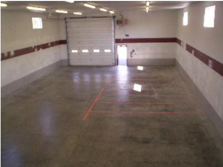
View of garage floor
