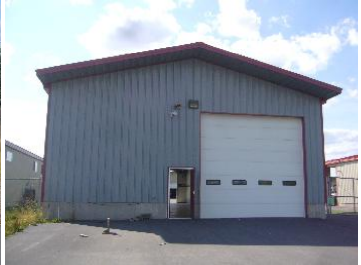
View of rear of building
