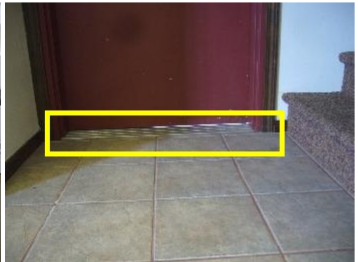
Air and light entering under and
