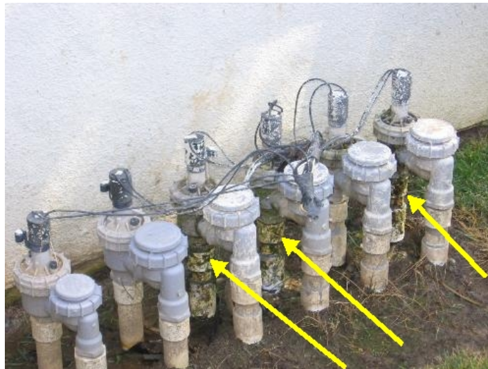
Visible leaking
