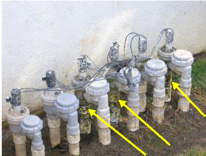
Visible leaking
