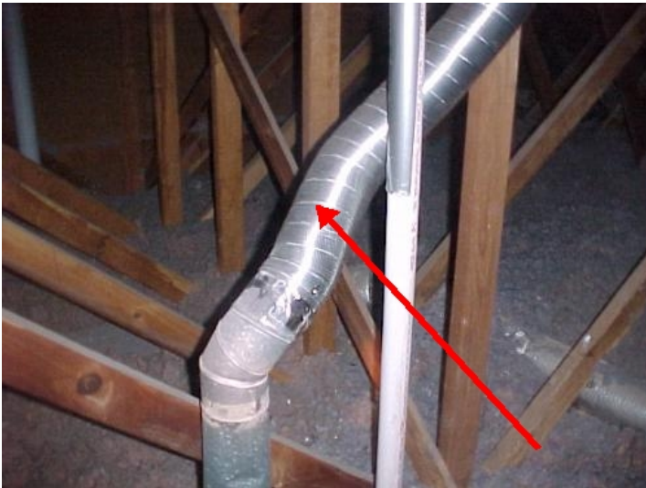
Improper dryer vent not exiting the interior of attic
