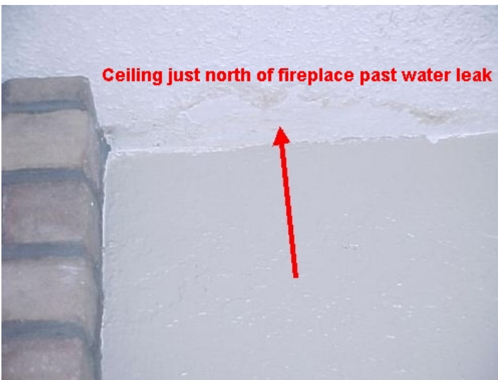
Ceiling just north of fireplace
