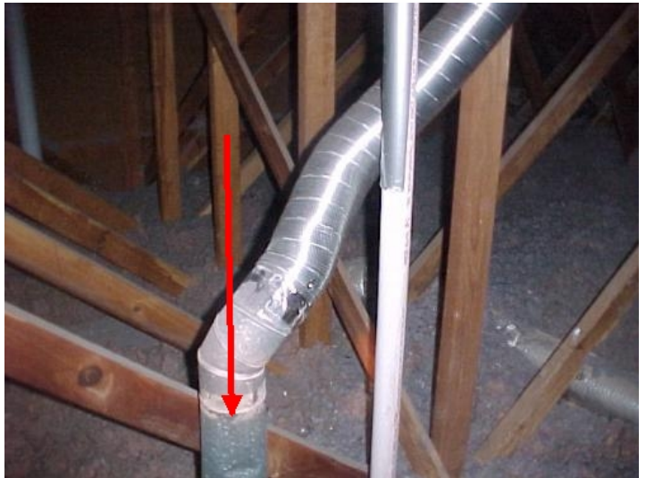
Dryer vent appears to be stopped up from arrow downward
