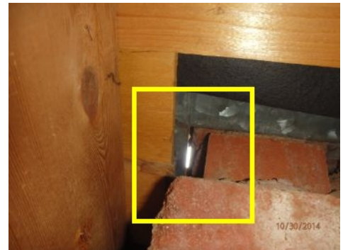
Visible light from inside of attic
