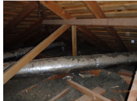
View of attic
