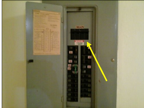
Main shutoff location: laundry room
