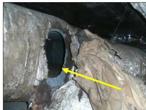
Disconnected ductwork
