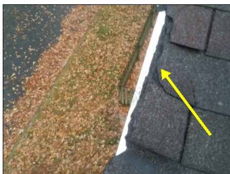
Shingle damage
