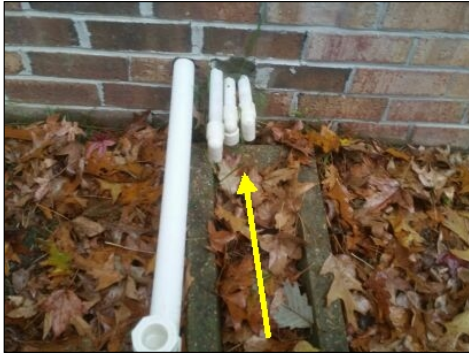
Recommend identifying the auxiliary line
