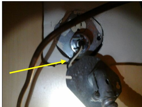
Exposed wiring
