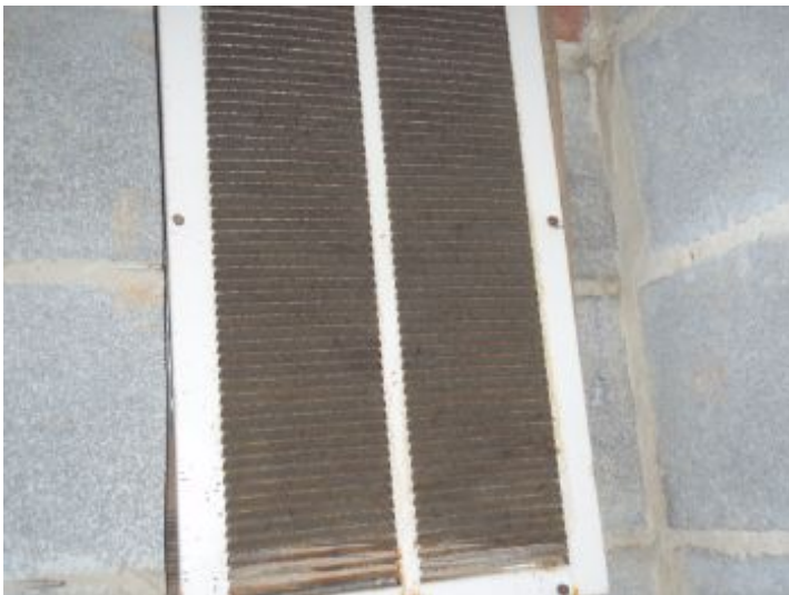
Vent opening under exterior entry stoop
